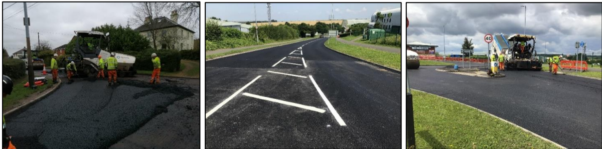
The programme of road resurfacing is improving the strength and surfaces of the county's road network.
